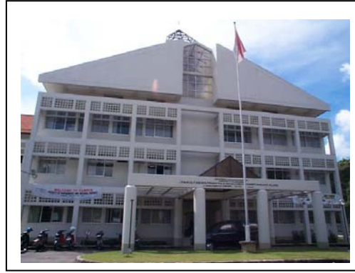
The newly constructed science faculty building
