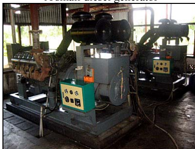
A small diesel generator
