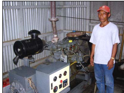
A small diesel generator
