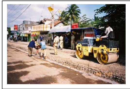
Repair work in progress on a national road in an urban area
