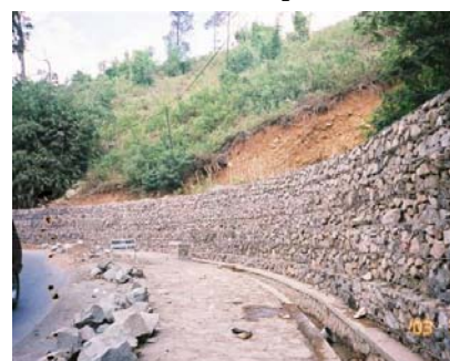
Figure 3: Site of a mudslide. 1000m 3 of sediments were removed using power shovels and dump trucks.
