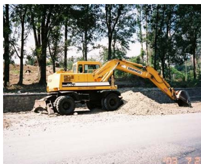
Figure 2: A DRU power shovel at work
