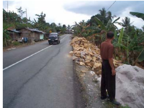
Figure 5: A vehicle driving over the center line on a cracked section of road slated for repair
