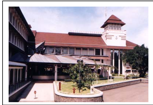
The new emergency unit built by the project
