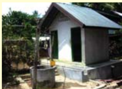
Mains water supply facilities
