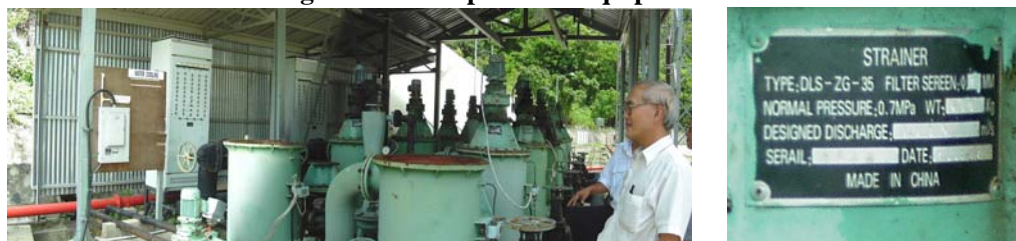
Figure 6: Silt Separation Equipment
