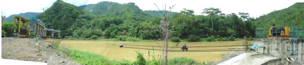
Figure 5: The Trash Boom
