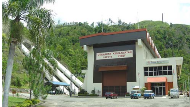
Entrance to Tenom Pangi Hydroelectric Power Plant
