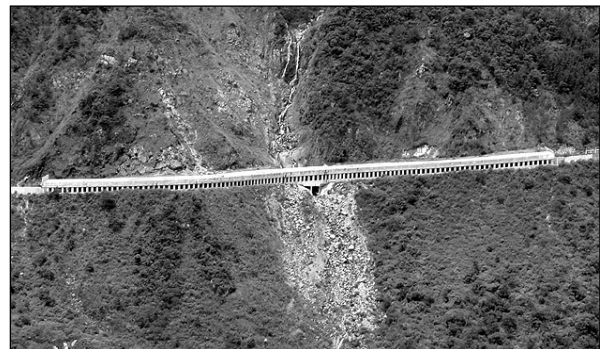
Photo 2: An aerial view of the rockshed
