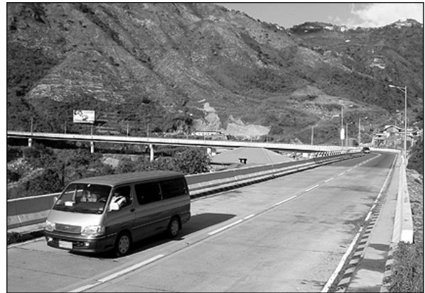
Target road (Badiwan Bridge on Pugo-Baguio route)
