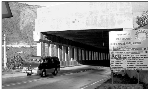
Photo 1: A rockshed on the Pugo-Batuio section
