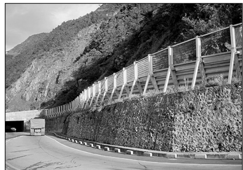
Photo 3: Fence for falling rocks in Tuba District
