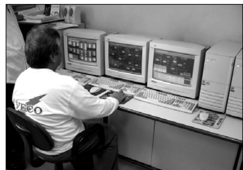
Photo 1: Terminals of SCADA System
