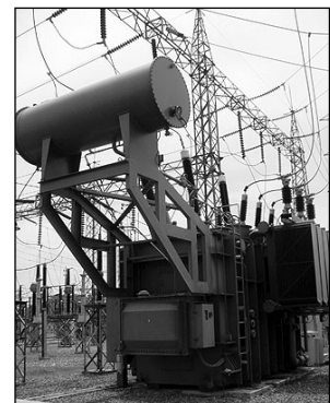
Photo: Newly installed transformer
