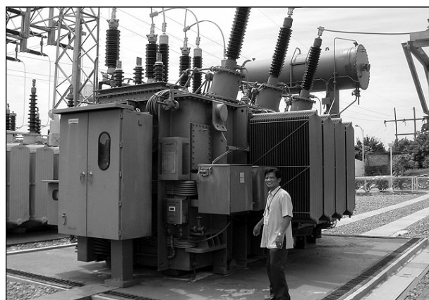
50MVA transformer installed at San Esteban Substation
