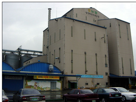
Livestock feedmill constructed in Haman under the project
