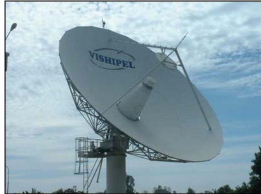
INMARSAT Land Earth Station (LES) in Hai Phong
