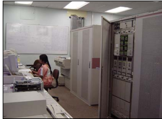
Switching Equipment at Kandy Switching Station of Sri Lanka Telecom
