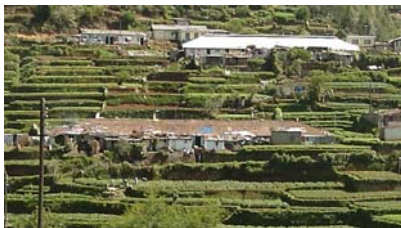
Reroofing of houses for plantation workers (The multiple dwelling house at the top has been reroofed and the one at the bottom has yet to be reroofed)
