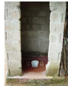
Lavatory for plantation workers
