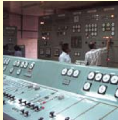
The control room of the power generator
