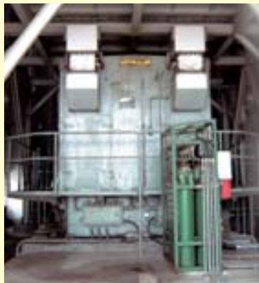
The power generator procured under the project
