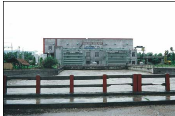
Power plant viewed from the lower reaches of the purpose-built channel
