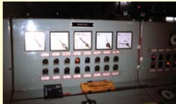
Power generator control room
