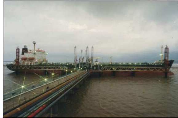
The No. 2 oil jetty constructed using project funds
