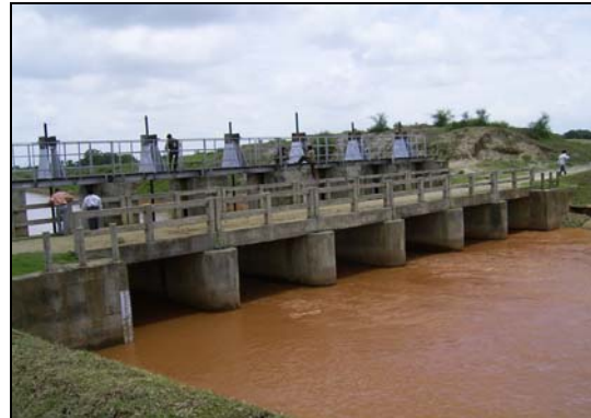
Indravati Main Canal
