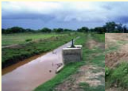
Indravati Irrigation Waterway
