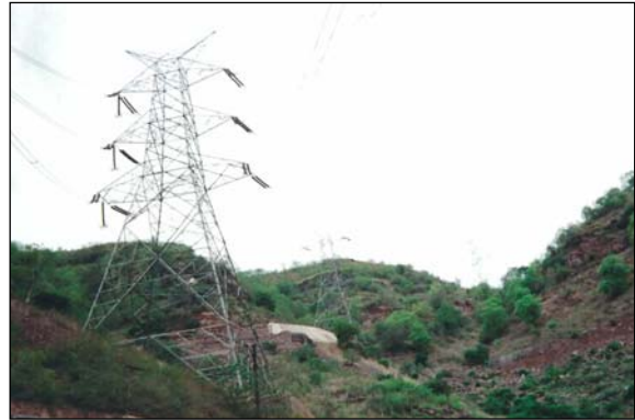
A steel tower and transmission lines constructed under the project
