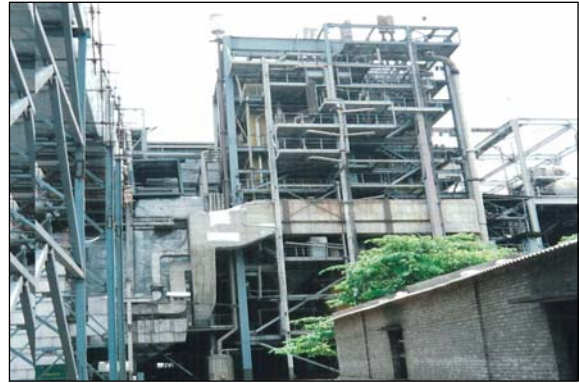
Overall View of Kothagudem “A” Thermal Power Station
