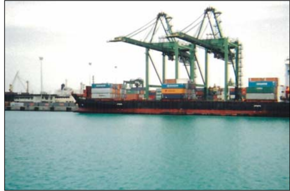
The harbor basin after dredging work was completed
