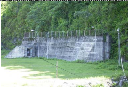
Entrance to the buried Mandu head works
