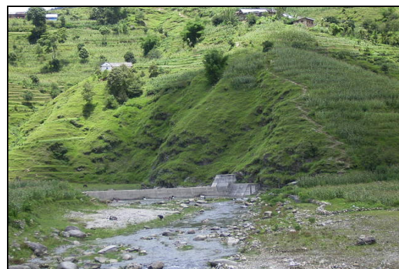
Erosion-Control Dam No. 5
