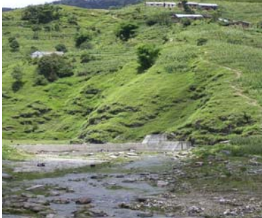
Erosion-control Dam No. 5
