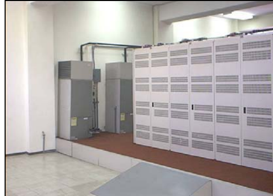
Switchboard at the Posmaqui Exchange
