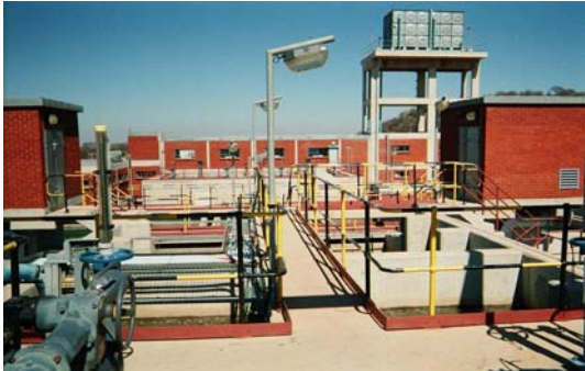
Mahalapye Water Treatment Works
