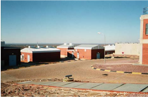
Mmamashia Water Treatment Works
