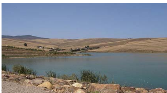
Hill dam in Khouithra
