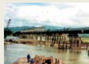
A bridge on Vietnam's Hanoi-Ho Chi Minh City railway: some sections are aging
