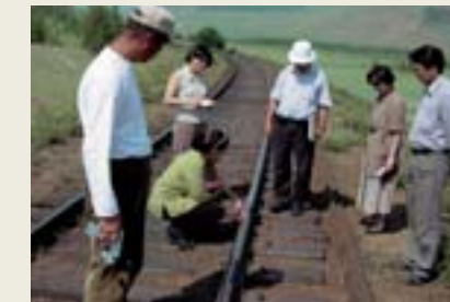
Highly durable surface-hardened track was laid under this project.
