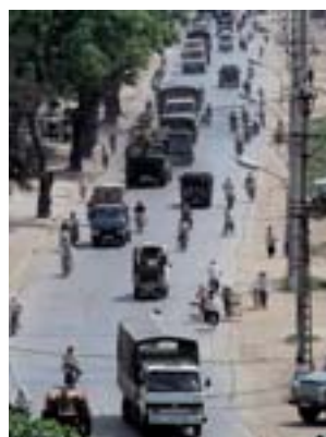
Highway 5 in northern Vietnam. It was constructed in one of the projects evaluated in "Impact Assessment of Transport Infrastructure Projects in the Northern Vietnam" that was reported on at the Shanghai Conference.
