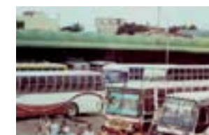
South Bus Terminal was constructed in 1992. The number of bus services was increased from 205 in 1988 to 250 in 1993 and to 335 in 2001. An average of about 15,000 passengers use Bus Terminal per day.
