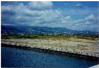
Photo 2-11: MCDP (3) Cebu City South Reclamation Project
