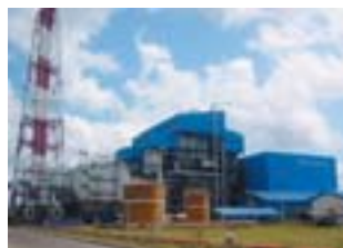
The Banjarmasin coal-fired steam power plant. This power plant is located in Kalimantan in the province of South Kalimantan and is an important power base for the region.
