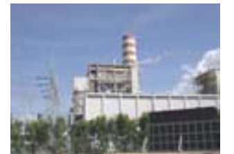
The Masinloc coal-fired power plant (300MWx2 generators) became operational in 1998; monitoring is undertaken on a regular basis.
