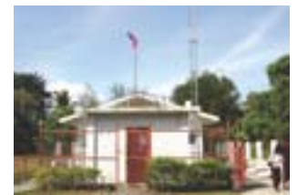
The environment monitoring station that was built near the Masinloc coal-fired power plant
