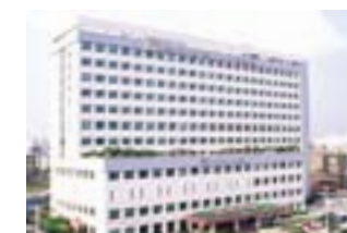
Seoul National University Hospital constructed with the ODA loan. It plays an important role as a medical facility, which provides advanced medical care.
