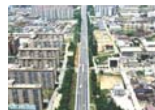
Highway constructed with the ODA loan has a considerable impact on the alleviation of congestion and on the physical distribution of traffic.
