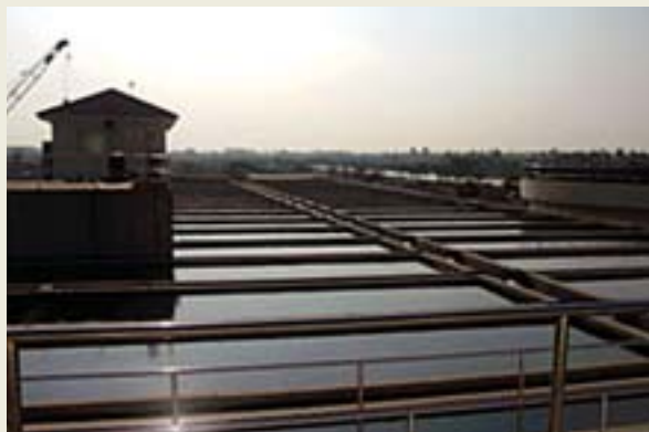
Maha Sawat water treatment plant constructed under the project
