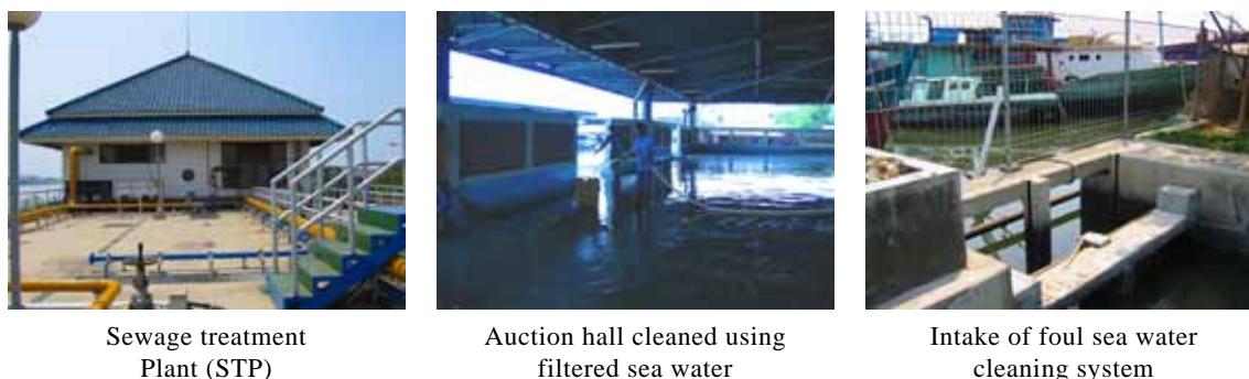
Figure 5: Facilities to improve sanitary and hygienic conditions of the port
