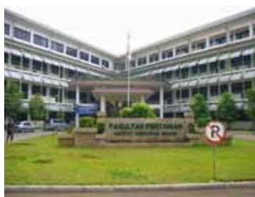
The newly-constructed Faculty of Agriculture building
