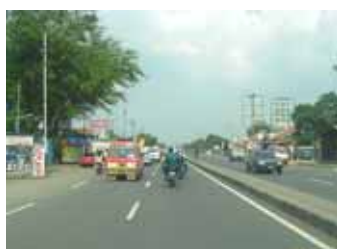
A section of road that was widened in central Bandung
