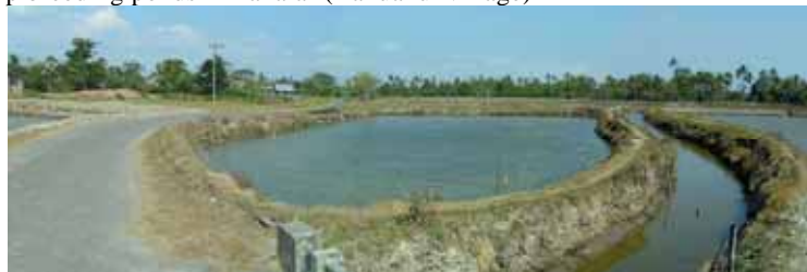
Shrimp breeding ponds: Roads and canals were rehabilitated
