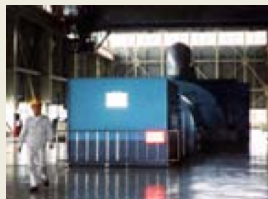
The boiler of the power plant
