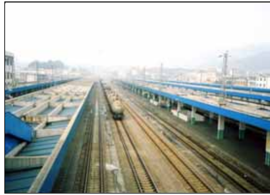
Huihua Station (the track on which the freight train is passing is covered by the project)
