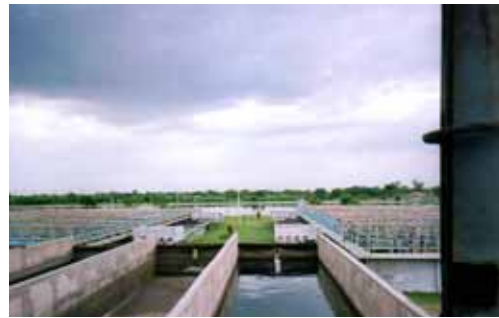
Sewage treatment plant built by this project
