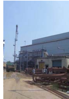
Figure 3: ESP* Equipment (Graphite India)
