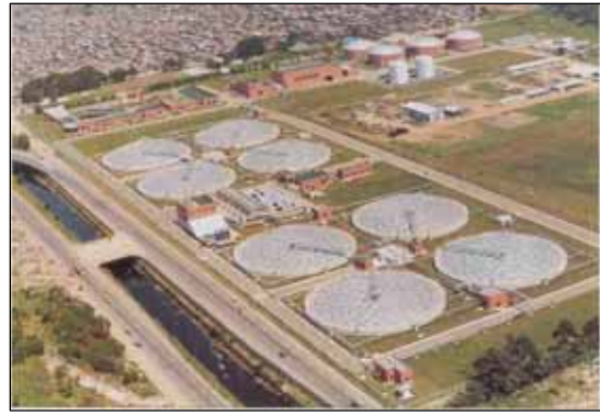
Aerial view of sewage treatment plant
