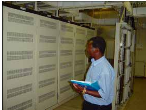
Switchboard at Bulawayo City Exchange
