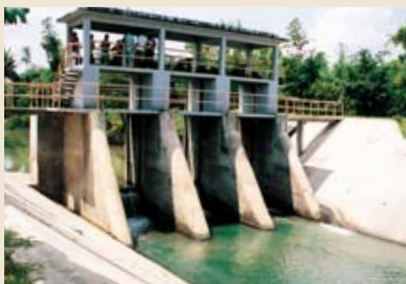
An irrigation sluice constructed through ARISP (Nabunturan, Compostela Valley Province). What I keenly felt once again when investigating this project is the power of irrigation facilities to achieve higher agricultural yields.
