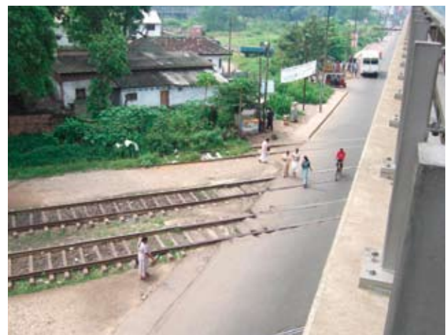
Viaduct over the railway
