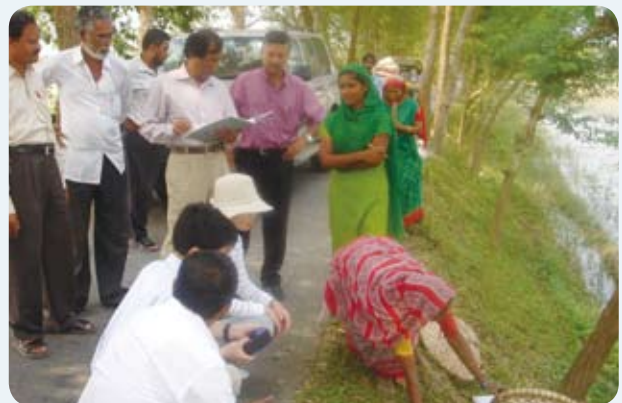
Female workers doing maintenance work of a rural road in the Great Faridpur Infrastructure Development Project
