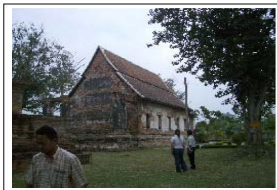
Site photograph: A renovated temple
