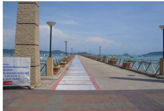
Tourist Dock constructed under the Project (Phuket)
