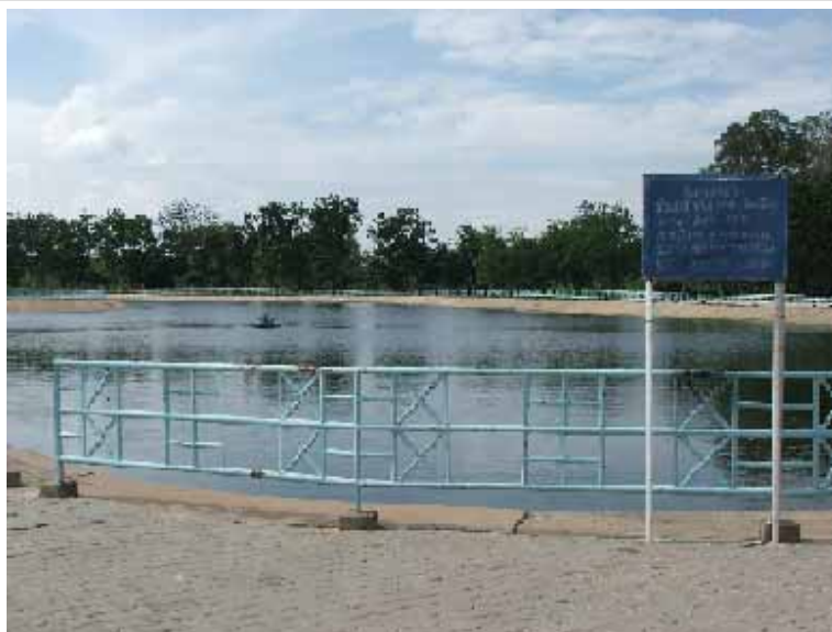
Huakhwang wastewater collection and treatment plant
