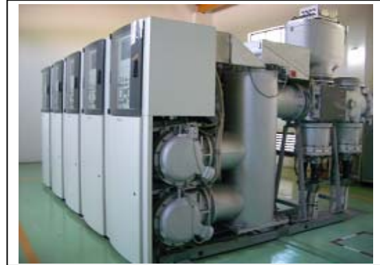
Site photograph: Substation equipment installed through this project
