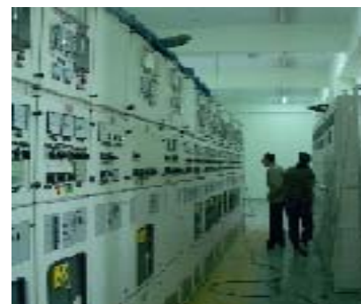
Photograph 1: Substation control board
